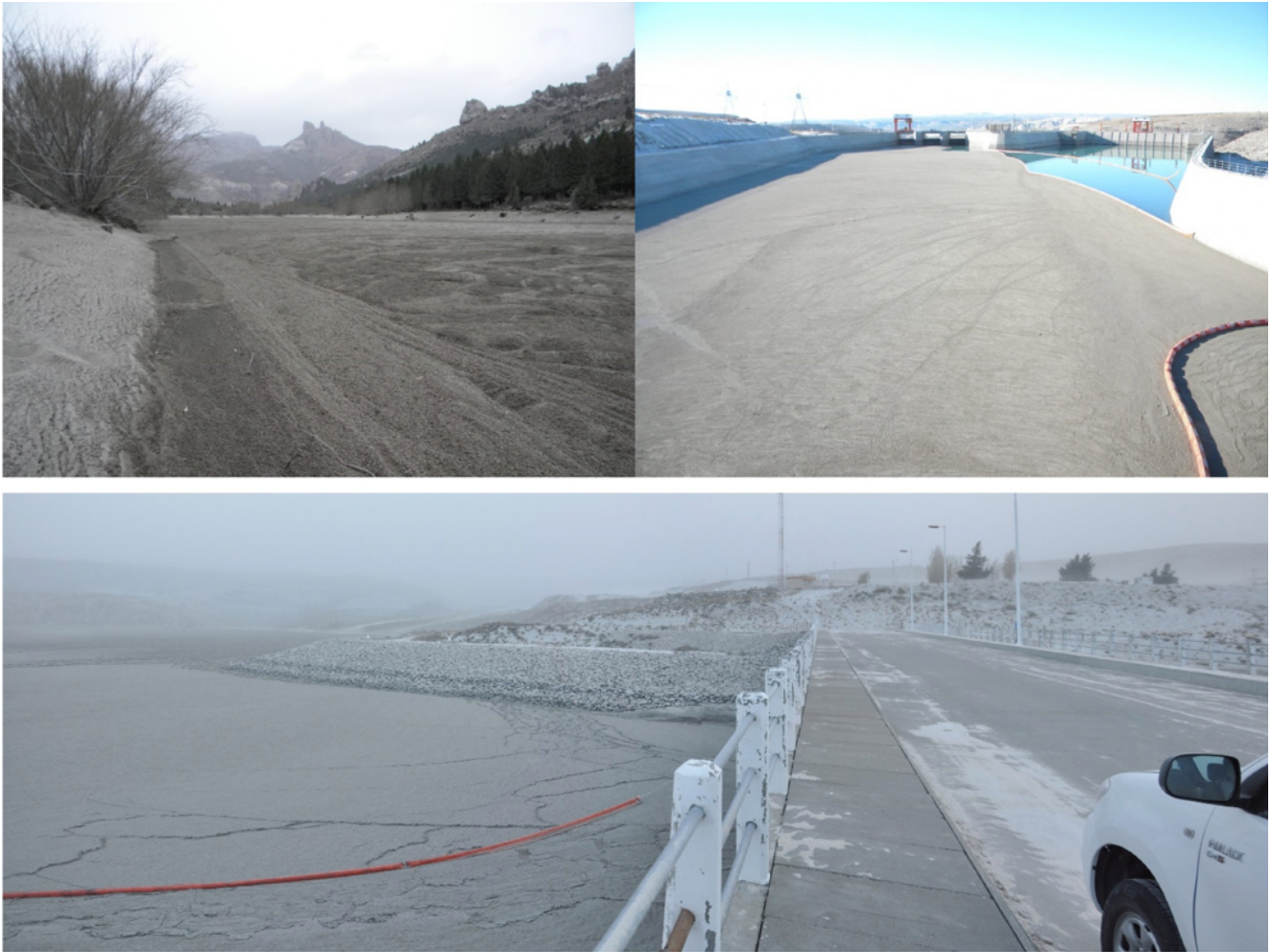
Figure 12: Drafting of floating pumice down the Río Limay during the 2011–2012 Cordon Caulle volcanic eruption, and lines of floating barriers attempting to halt and divert away pumice rafts close to the Alicurá power dam during the first days of the eruption (below) and the following weeks (at the top right).
