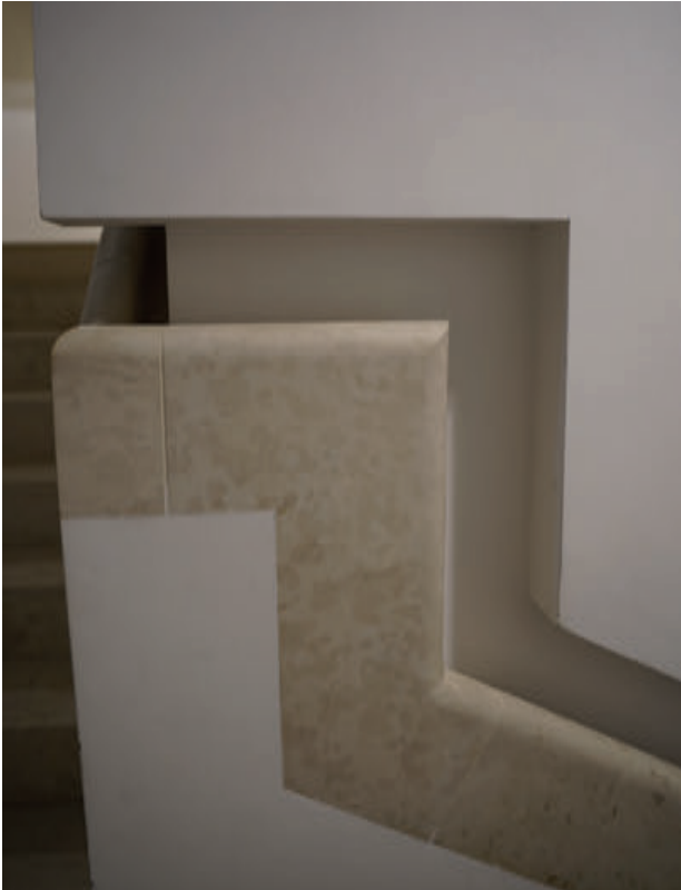
Figure 11 | R. Rizzi, The Shakespearean theatre in Gdańsk, 2005-2014. The stone handrail of the interior staircases as guise of the rogge, small artificial water canals. Photo: Adam Garstka.
