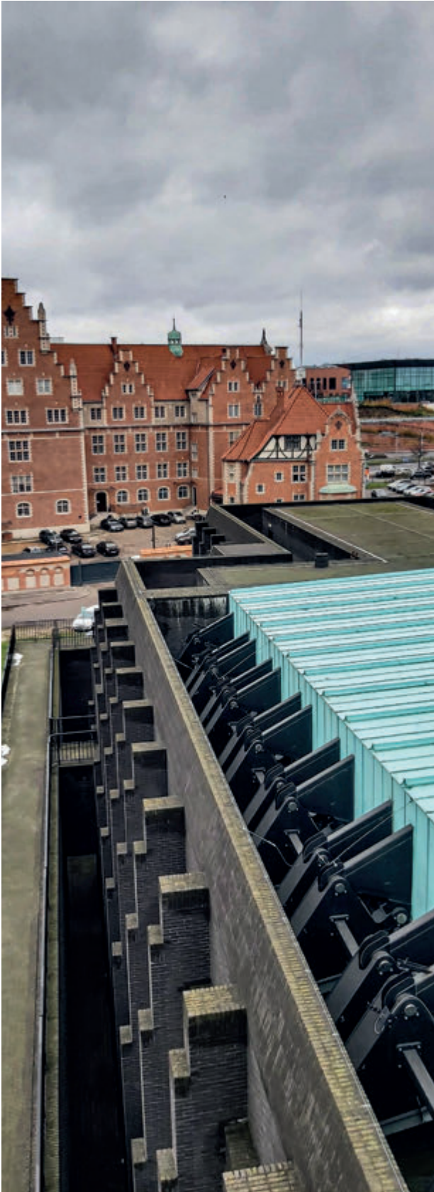
Figure 6 | R. Rizzi, The Shakespearean theatre in Gdańsk, 2005-2014. Technological detail of the closed roof. Photo: Bahaa Bou Kalfouni.
