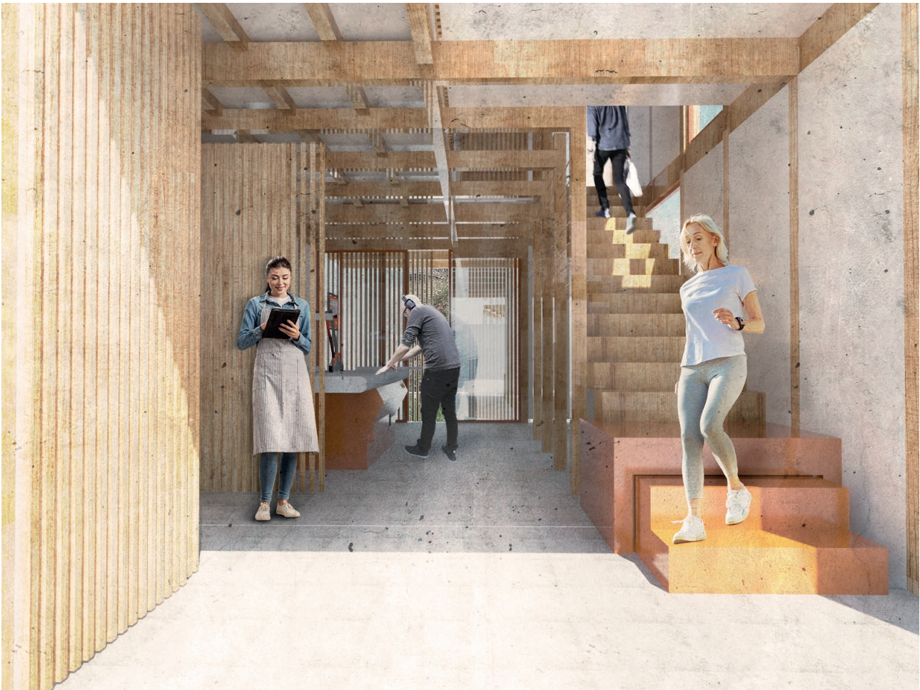
Figure 10 | Visualisation of the interior of the carpentry woodworking workshop with its wooden frame construction and eucalyptus boards wall enclosures; author M.Orszt.
