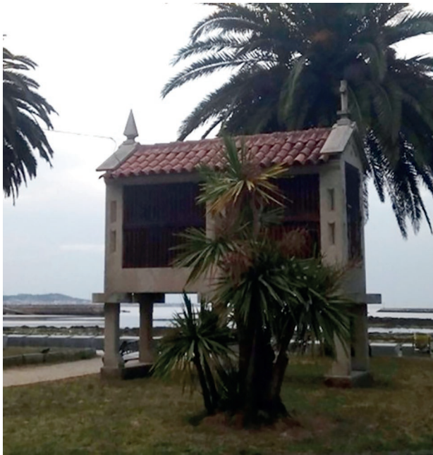
Figure 3 | Stone construction of a granary with wooden details, Cambados, fot. M. Orszat.
