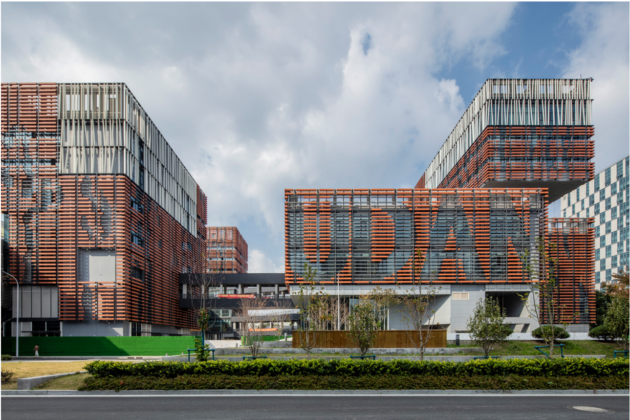
Figure 3 | Fudan Campus Business School. Shanghai, China (under construction). Photo: Shen Zhonghai.
