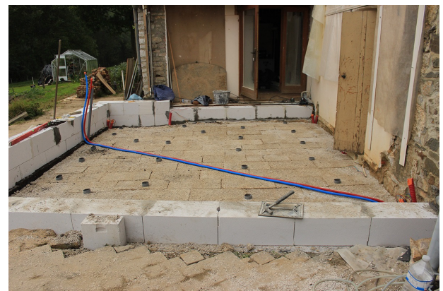
Figure 4 Floor isolation with hempcrete blocks and no adhesive agent in a detached house (iso hemp.com)
