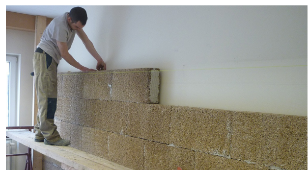
Figure 5 Acoustic interior insulation with hempcrete blocks for a school renovation (iso hemp.com)
