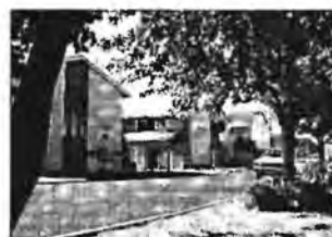
a) The orientation of residential blocks away from the public realm (in this case the street) inhibits passive surveillance over the street
