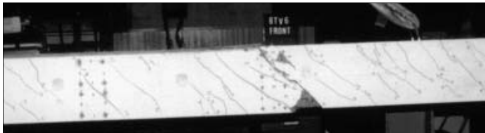
Figure 14c. Computed and observed crack development in the front web (BTV6)
