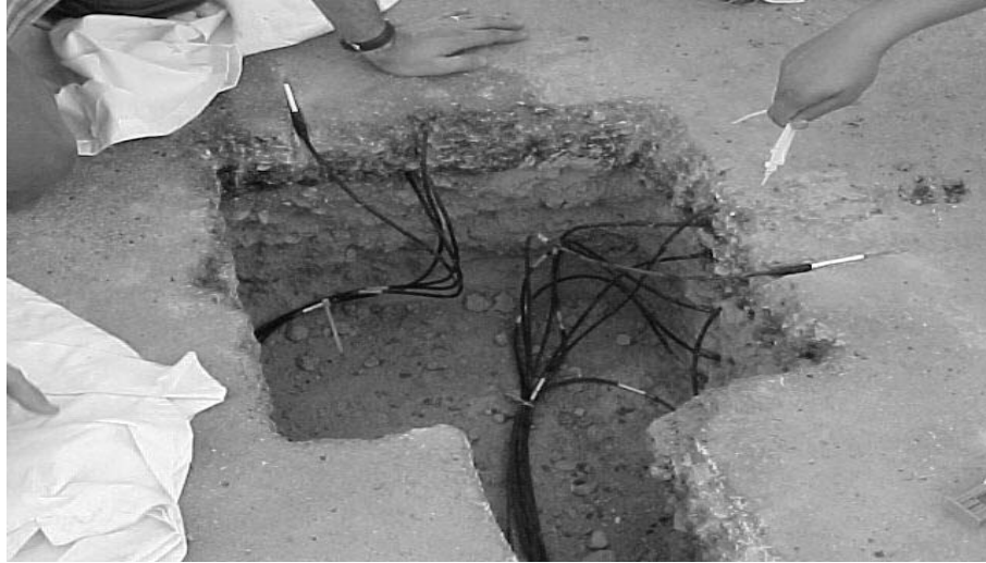
Figure 1. Installation of thermistors
