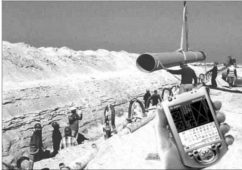
Figure 4. King Faisal University Construction Site (the foreman's equipment)
