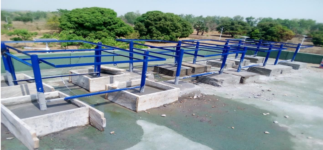
Figure 4: Installation of metal structures
