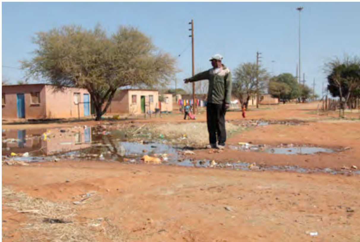
Figure 6 At the intersection of Kangulu Street in Platfontein's Xun area water is still dammed up, despite a recent water pipe repair operation. Motorists and pedestrians are unable to pass safely through the area (Photograph: JWN Tempelhoff)
