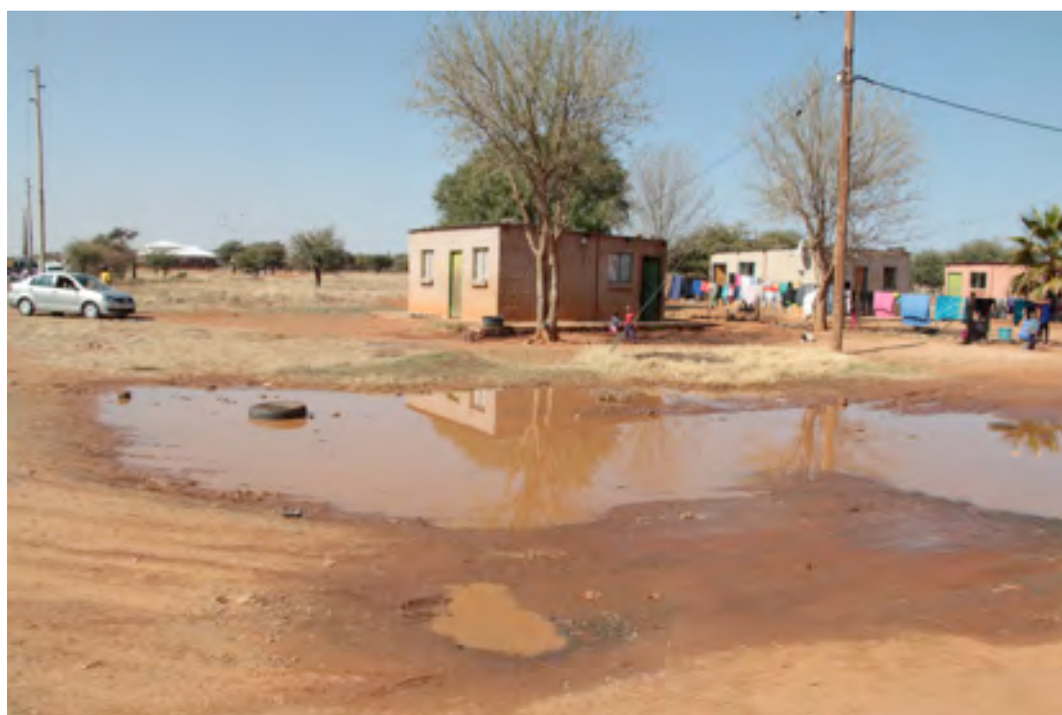
Figure 9 A pipe leak at a T-junction into Kamatoka Street, the main road of Platfontein. In the rainy season the nearby houses are frequently flooded causing significant damage to residents' domestic belongings (Photograph: JWN Tempelhoff)
