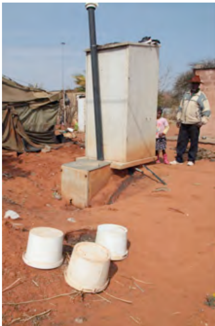
Figure 8 Out of sheer desperation this toilet has a pipe extension for raw sewage to run down in a hole adjacent to the toilet bag container. In the foreground are a number of plastic containers for faeces that are emptied into the hole at the back (Photograph: JWN Tempelhoff)
