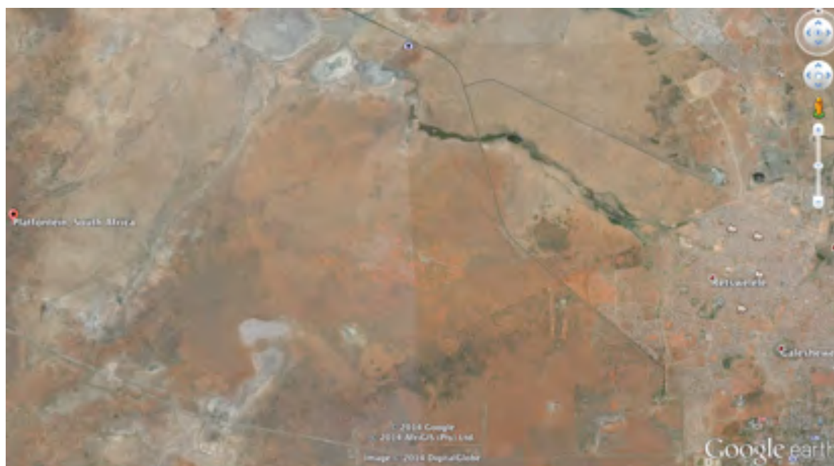
Map 5 Satellite image showing the dark line of raw sewage emanating from the Gogga Pump station – the largest wastewater treatment works in the Kimberley area. The highly dangerous spill is on the communal property of the San at Platfontein (Google Earth)
