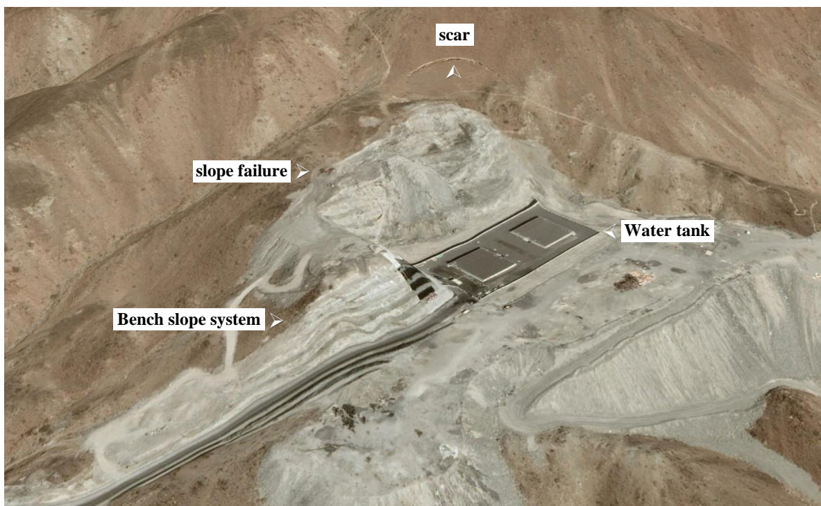
Figure 2. Landsat Google image (20 Mar 2021) showing the water tank and slope failure above it.
