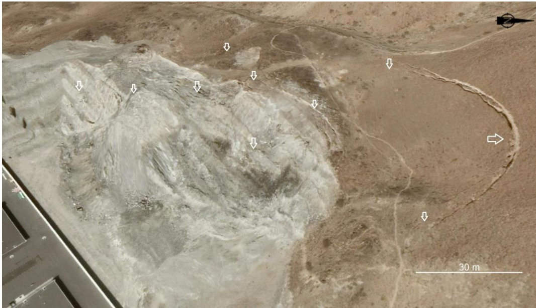
Figure 7. Collapse of benches initiating large fractures parallel to the main slide area.
