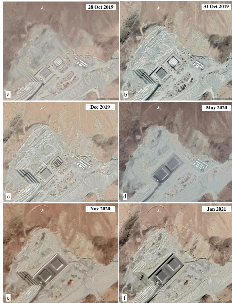
Figure 8. Satellite images (a-f) show that slope failure started between 28 and 31 October 2019 (a and b) as a result of major slope excavation and removal of the toe support in order to construct the tank.
