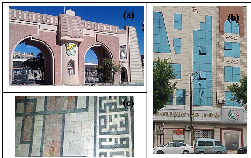
Figure 4. Examples of usage of tuff as (a, b) outside covering stone; (c) Decorative stone.
