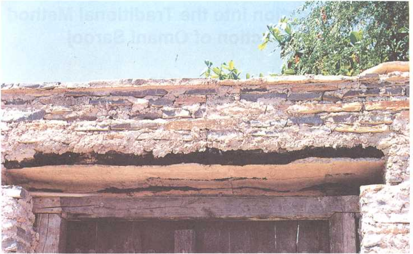
Figure 1. Use of sarooj in buildings.
