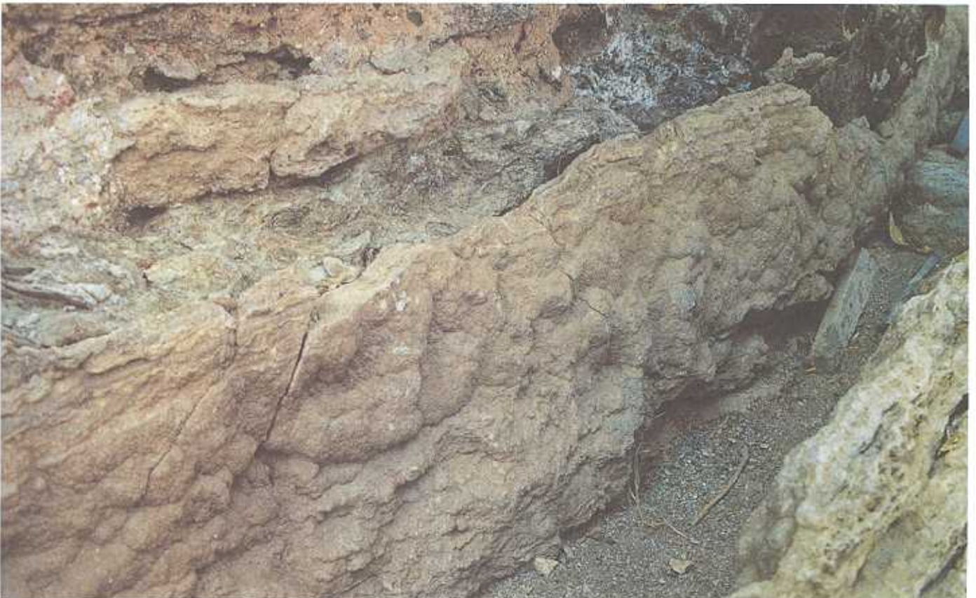
Figure 4. Sarooj used in lining Aflaj channels (Hammam Falaj in Boshier).
