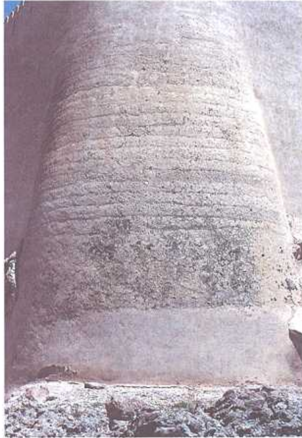
Figure 2. Sarooj used in building Kisra tower in Rustaq castle of sarooj in buildings.
