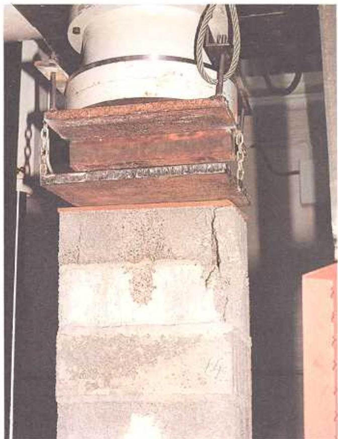
Figure 18c. Failure of a tested column.
