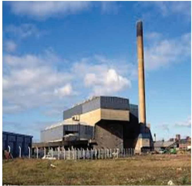
Figure 1: Eastcroft Incinerator in Nottingham
