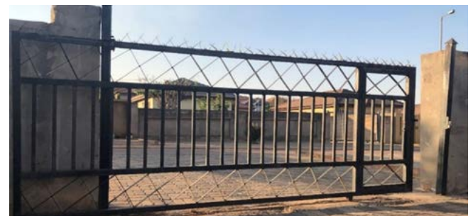
Figure 1. An example of a non-motorised sliding access gate in a semi-suburban home
