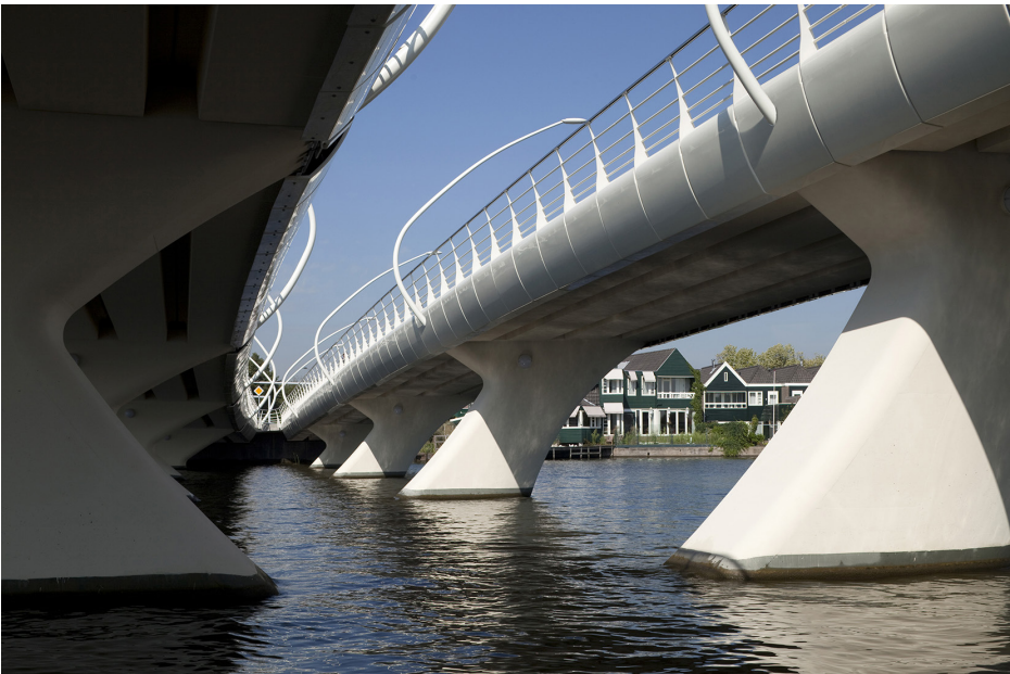
Figure 9 Pedestrians and cyclists have a bridge of their own. A void separates them from motorised traffic (source: Joris Smits)
