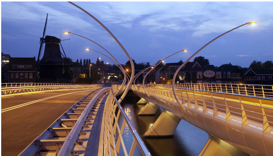
Figure 13 Light masts define the space and viewing directions. They emerge from the void in order not to obstruct the outward view (source: Joris Smits)
