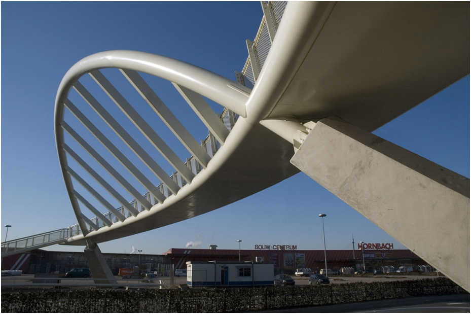
Figure 4 The pedestrian bridge in the Zuidelijke Randweg, 2005 (source: Joris Smits)
