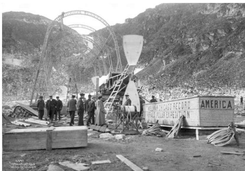
Figure 7 The hangar and airship under construction, Virgohamna, 1906. The person standing in front of the propeller blade is most likely Walter Wellman. (Courtesy Norwegian Museum of Cultural History [Norsk Folkemuseum].)
