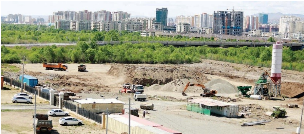
Figure 4. Floodplain erosion of Tuul River
