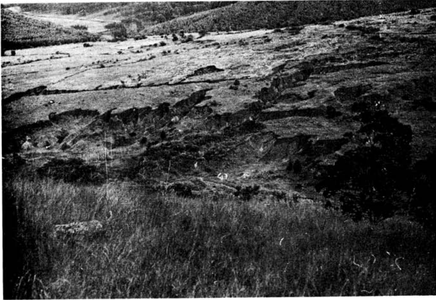
Fig. 7. Deep erosional dongas, characteristic of lower mountain slopes in Mlilwane South.
