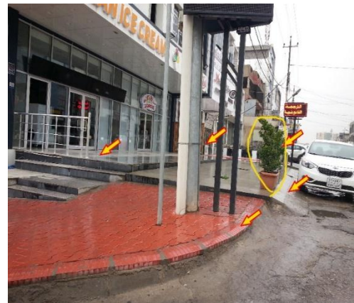
Figure 11. Poor building entrance design and building and landscape elements configurations.
