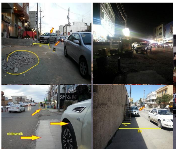
Figure 13. Poor lighting condition of some parts of the street.
