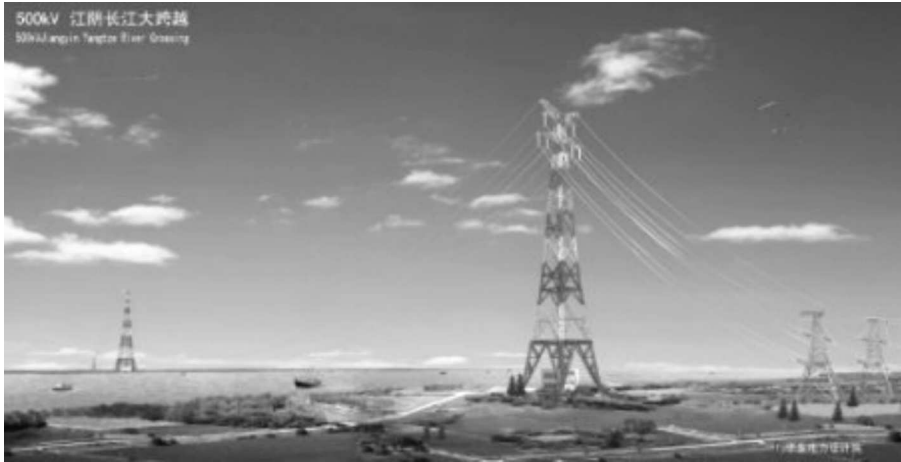
Fig. 1. 500kV-powerline section running over the Yangtze River (the People's Republic of China)
