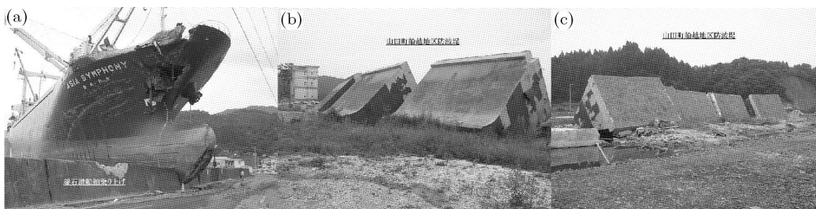
Fig. 11. (a) Piled-up ship on bank at Kamaishi Harbor, (b) breakwaters turned over counter-clockwise at Yamada-Cho, (c) breakwaters turned over showing bottoms at Yamada-Cho (courtesy of Mr. I. Teranishi)
