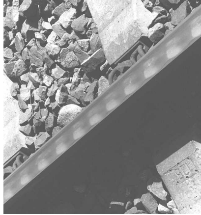
Fig. 1. View of a track segment with the corrugated rail (slip waves)
