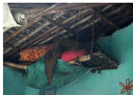
Fig. 6: Households Tie their Belongings to the Rooftop of the House
