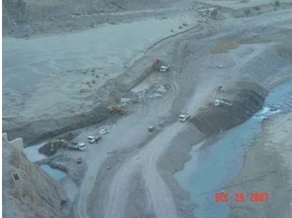
Fig. 2. The construction site in its early stage.
