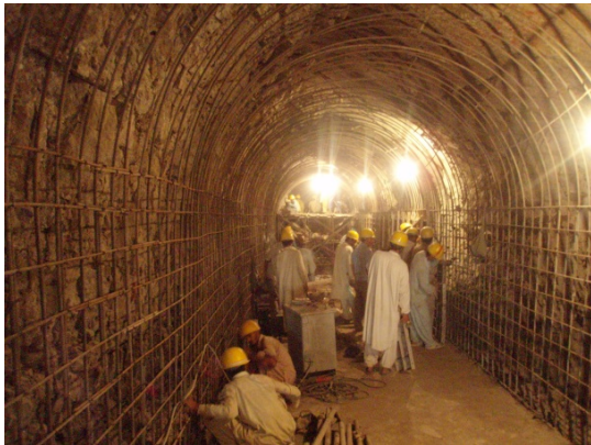
Fig. 5. Additional concrete lining preparation for the adit of the tunnel.
