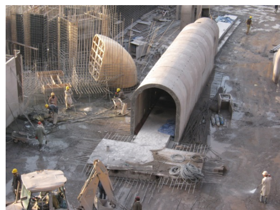
Fig. 7. Formwork for power intake and precast concrete gallery.
