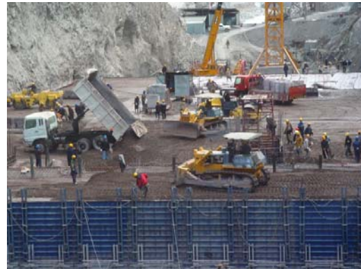
Fig. 4. Placement of roller compacted concrete.
