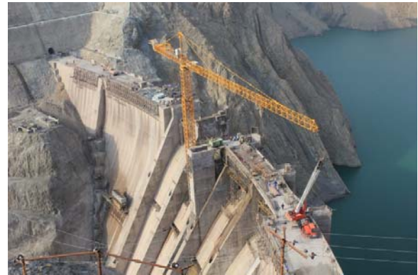
Fig. 8. Airscape view of the dam during construction.
