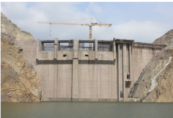
Fig. 9. Upstream view of the dam.
