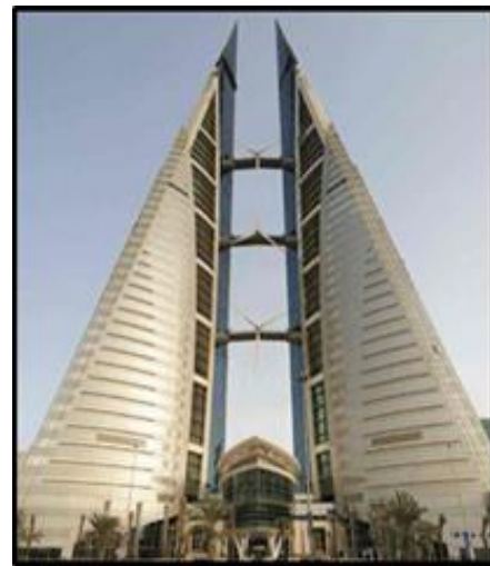
Figure 8 Bahrain Trade Tower project
