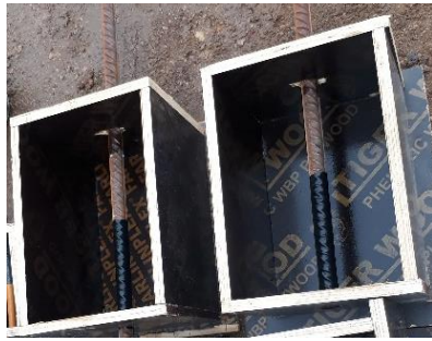
Figure 3. The final composition of the block moulds with their steel reinforcements
