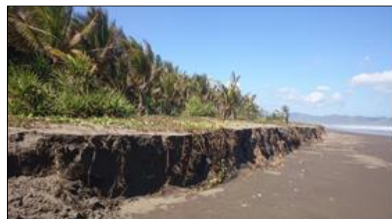
Fig. 12. Abrasion of the alluvium deposits in the Nusawungu Coastal Area which has occurred due to the sea water waves (source: personal documentation).
