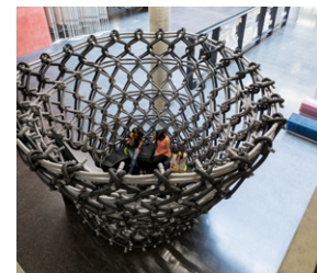
FIG. 3 Foamed fabric sleeves: Lightweight experimental pavilion FFin, © 3a FFin, © 3b Tobias Etzer.
