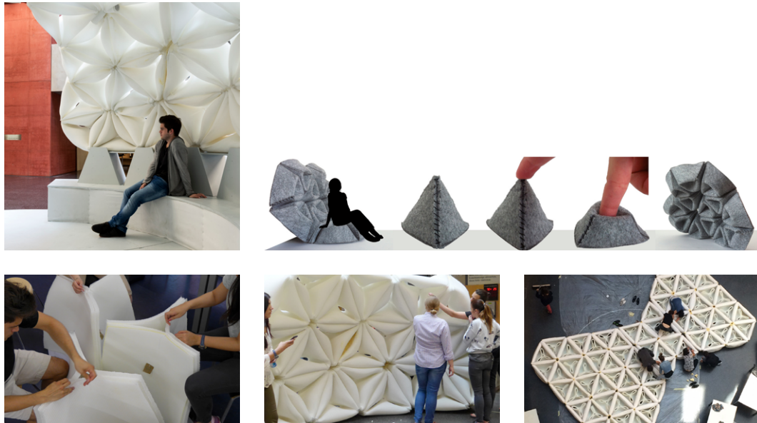
FIG. 8 Experimental pavilion: Modular system made of folded, foamed spacer fabric elements, © FFin.
