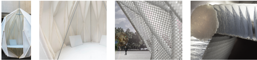
FIG. 5 Fully-fashioned structure, folded foamed spacer fabric, FFin © 5a+b Christoph Lison, Fig 5c-d, Mock-up and detail, © FFin.
