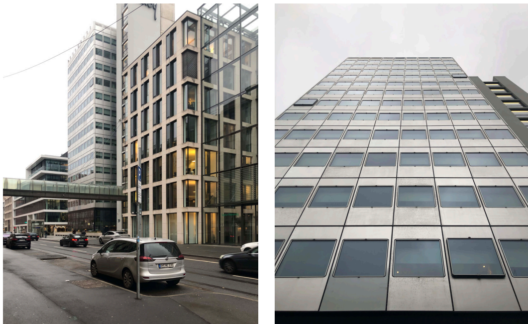
FIG. 6 The former Commerzbank high-rise after the recent upgrade and conversion, 21.11.2021. Photos: Rouven Grom
