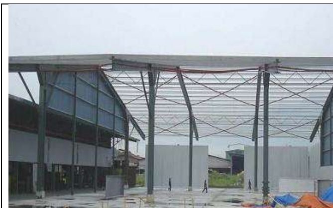
Fig. 22: Wilson Hall during the construction [74]
