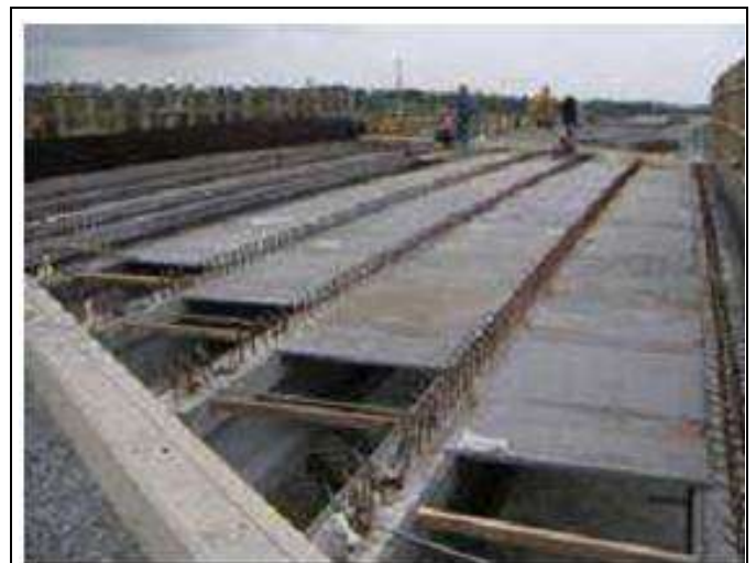
Fig. 7: Bourg les Valence Road Bridge, France
