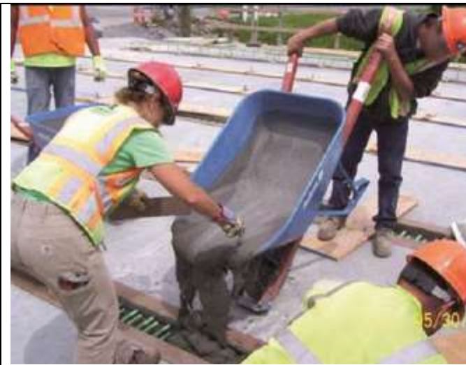
Fig. 12: Longitudinal connections cast between deck-bulb-tee girders on Route 31 Bridge in Lyons, New York
