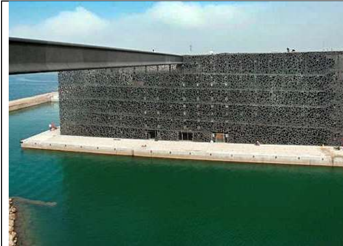
Fig. 24: Mega project: MuCEM with UHPC lattice facade, roof and footbridge.
