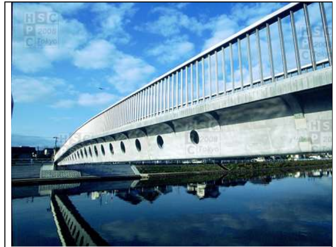
Fig. 6: The Sakata-Mirai footbridge in Japan
