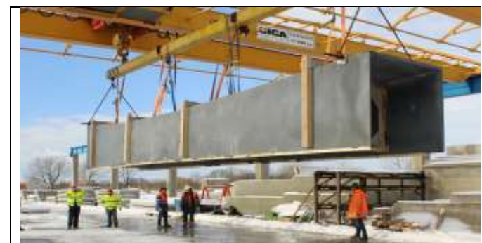
Fig. 17: Transport of final 1:1 mock-up of the footbridge in upside-down position
