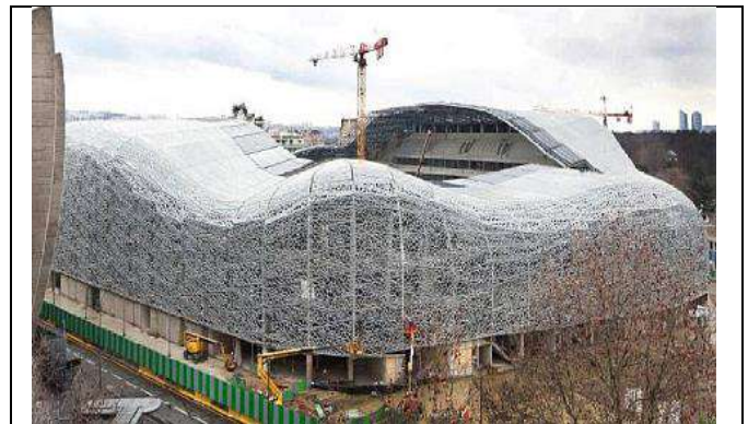
Fig. 23: Stade Jean Bouin, open lattice façade allowing sunlight to filter through
