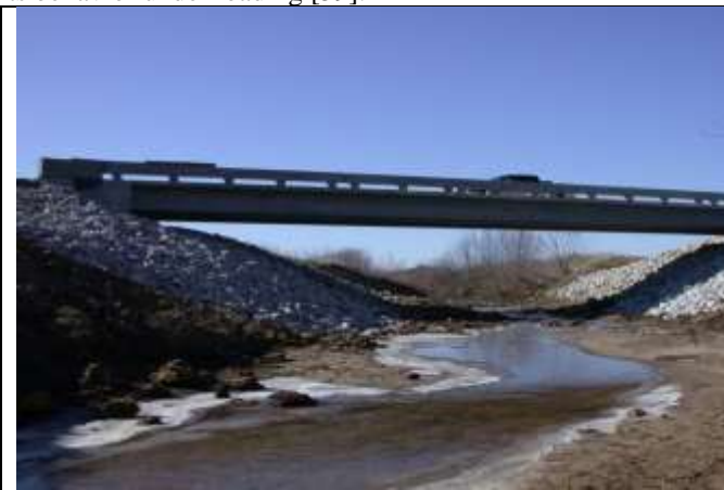
Fig. 9: Mars Hill Bridge in Wapello County, Iowa
