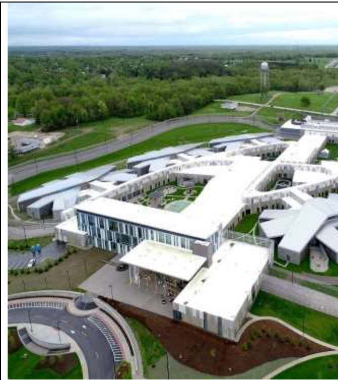
Fig. 26: Fulton State Hospital, Fulton, Missouri, USA
