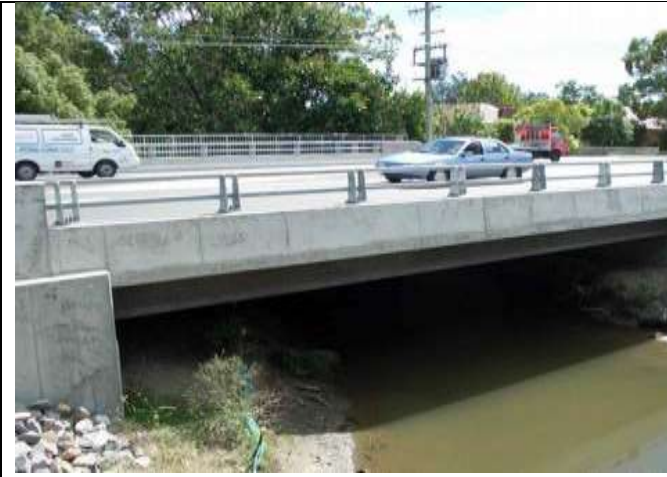
Fig. 8: Shepherd Creek Road Bridge in New South Wales, Australia.
