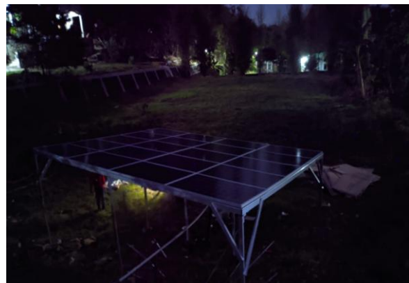
Figure 3. Solar panel installation using 20 panels
