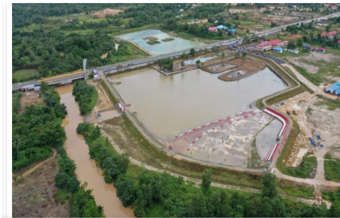
Figure 7. Flood Management in Wanggu Watershed with a Retention Pond
