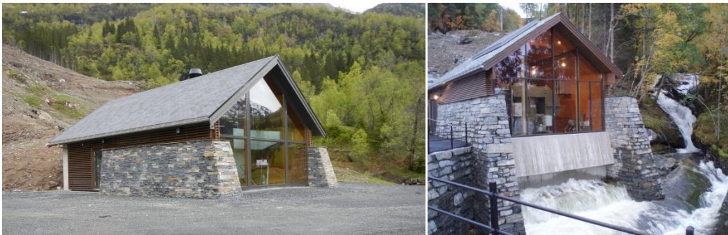
Figure 2. Two private small hydropower plants in Norway: Vassvik 3.100 kVA (left), Ytre Alsaker 5.490 kVA (right) (Source: Småkraft AS http://www.smaakraft.no/ )
