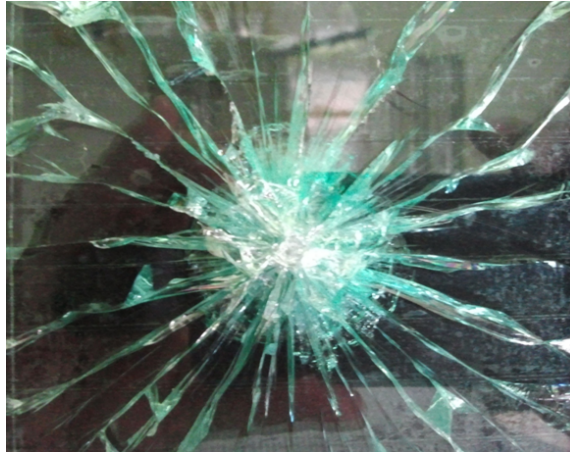
Fig. 4: The damage and failure of glass plate subjected to copper projectile at a velocity of 71 \text{ ms}^{-1} .
