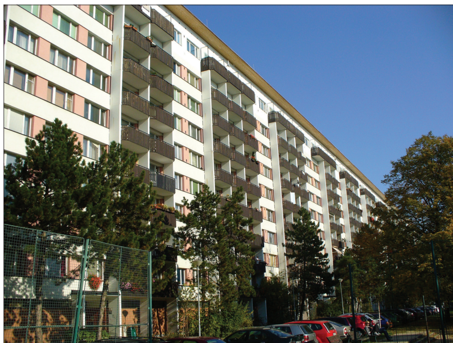
Photo 1. Characteristic high-rise building at Lesná. The balconies are new "components" appeared only after 1990. (Photo by ANDRÁŠKO, I.)
