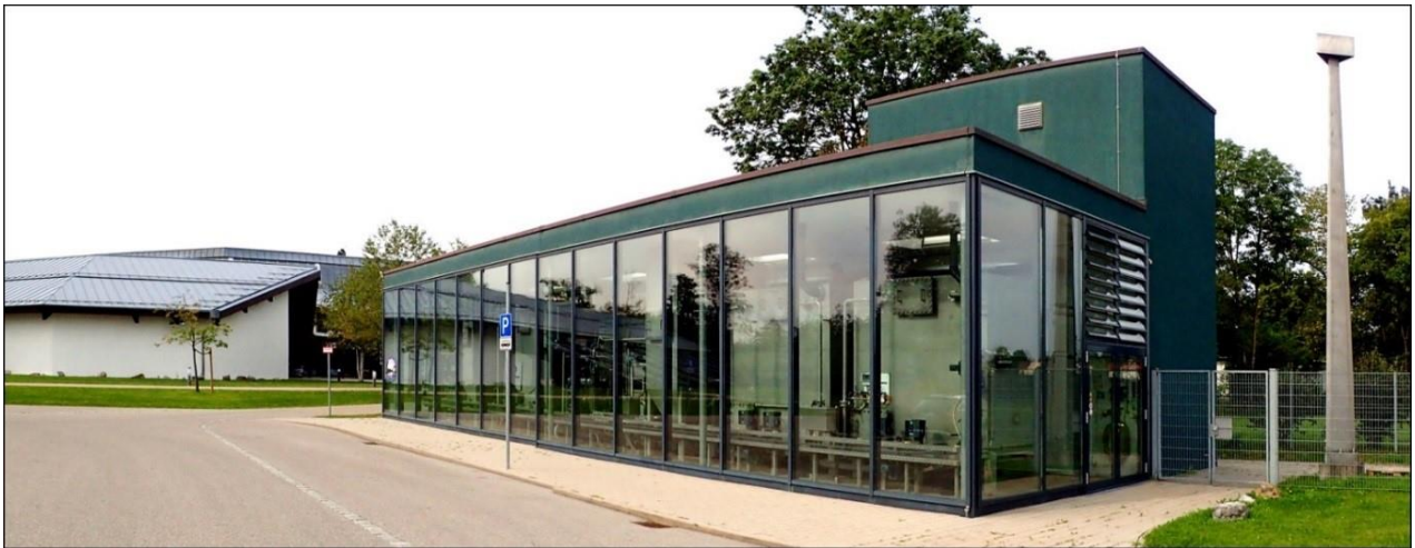
Figure 7. The building housing the borehole used to extract mineral thermal waters in Bad Aibling. The building is located near the entrance zone of the health resort and makes it possible to observe the mining process of groundwater extraction
