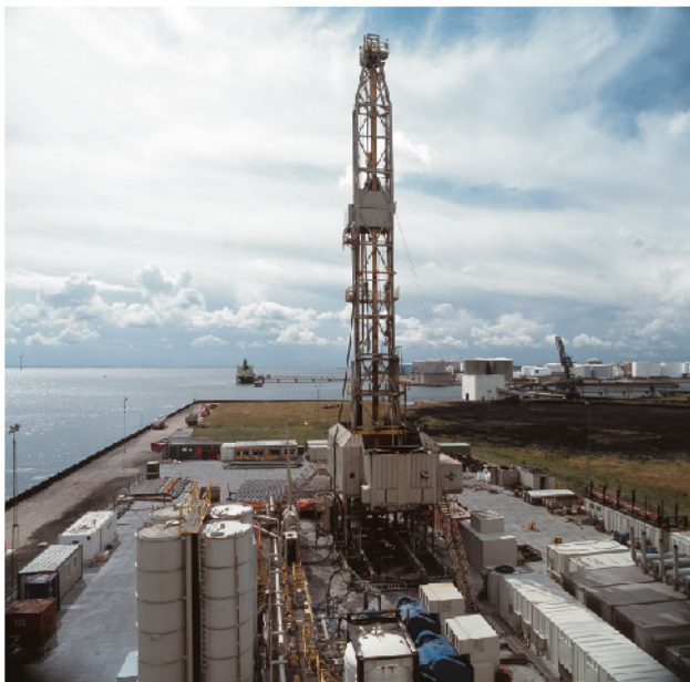
Fig. 3. The drilling of two deep wells at Margretheholm, central Copenhagen.
