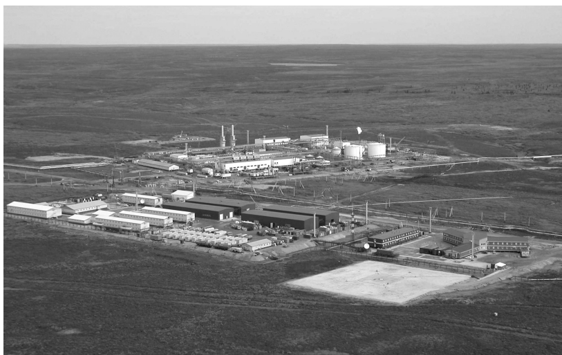
Figure 3. Oil production facilities, storage halls, heliport in front and accommodation complexes in South Shapkino. Crude oil production is estimated to reach 6800 tonnes per day by the end of 2004. Photo: Fortum Oil and Gas Oy.
