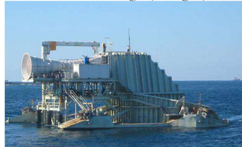
Fig.7. Off-Shore oscillating water column unit
