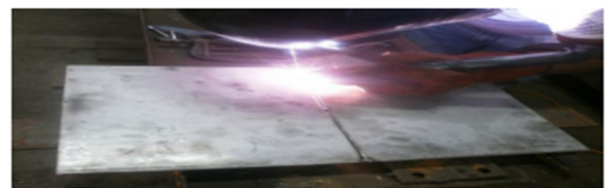
Fig. 1. Arc welding of steel plates
