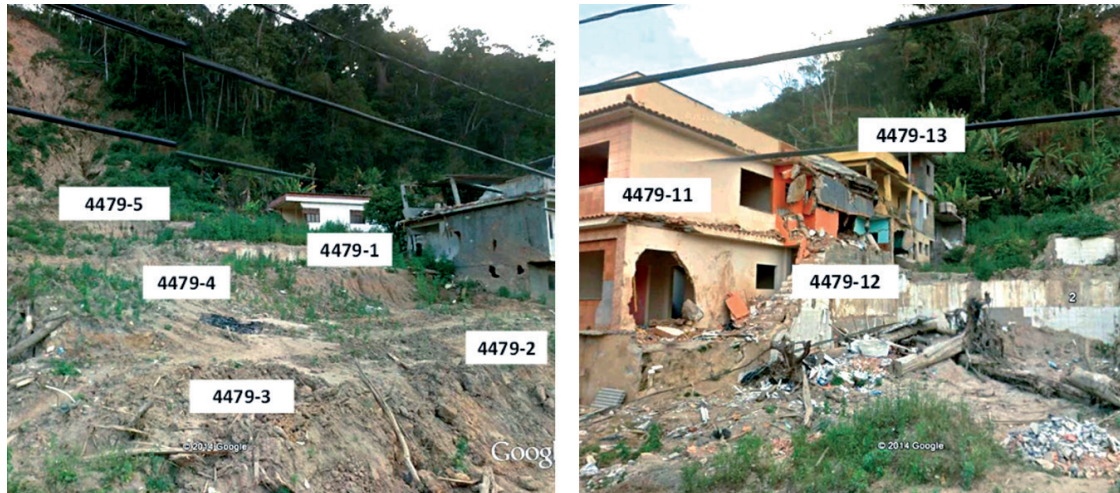
Figure 9. Floor view of buildings 1, 3, 4, 5, 11, 12 and 13 damaged by the landslide 4 479, acquired using Google Street View.
