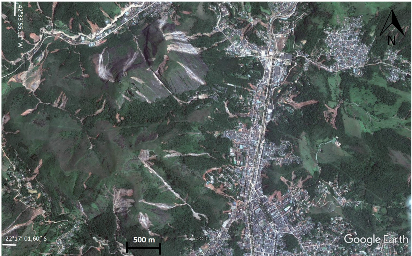
Figure 5. Aerial view of urban landslides in the municipality of Nova Friburgo.
