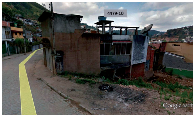
Figure 10. Floor view of the building 10 that was damaged by the landslide 4 479, acquired using Google Street View.
