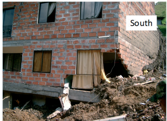
Figure 23. Photographs of the landslide pathway and three buildings that were partially destroyed by the El Socorro landslide.
