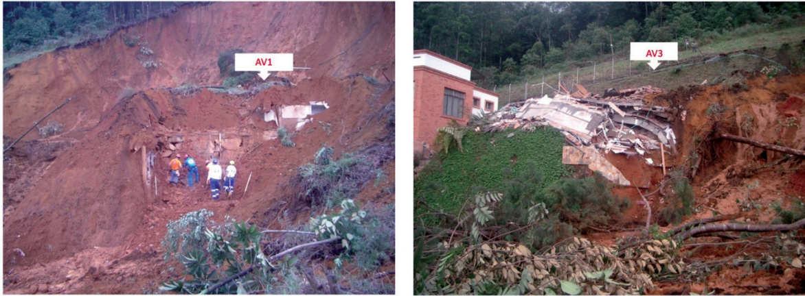
Figure 27. Photographs showing the damage to houses AV1 and AV3 during the Alto Verde landslide.
