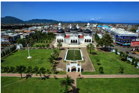
Figure 2. Baiturrahman Great Mosque Before Renovation with Green Open Space. Source: YR's Photo, Informant Collection (2015)
