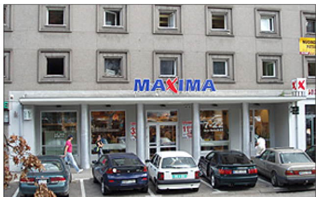
Fig 10. Shop Maxima in the multi flat house in Vilnius, A. Smetonos st. (Shop... 2013b)
