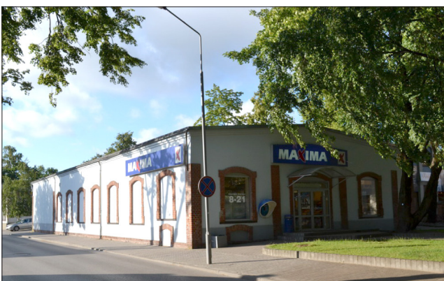
Fig 8. Shop Maxima in existing building in Šilutė. (Shop... 2013)
