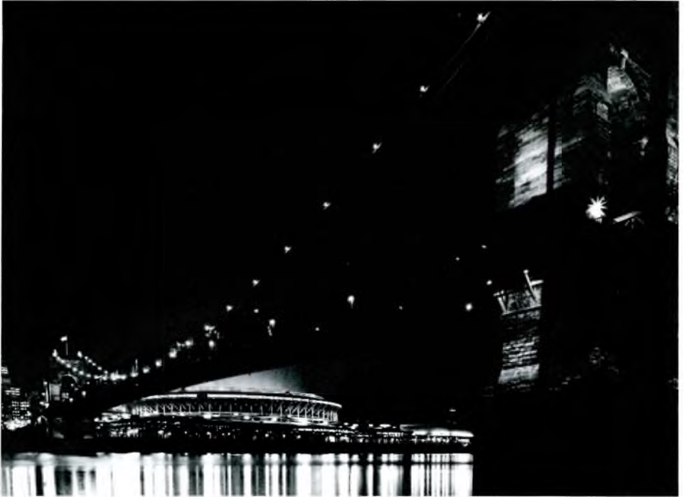
The graceful span of the John A. Roebling Suspension Bridge is a contrast of Old World charm against the skyline of downtown Cincinnati.
