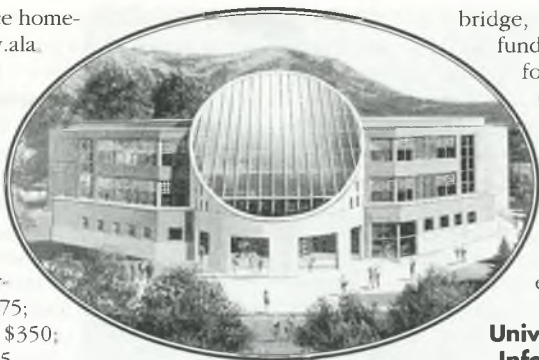
Southern Utah University's new library features a two-story reading room that offers library users a 50-mile view of the valley.
