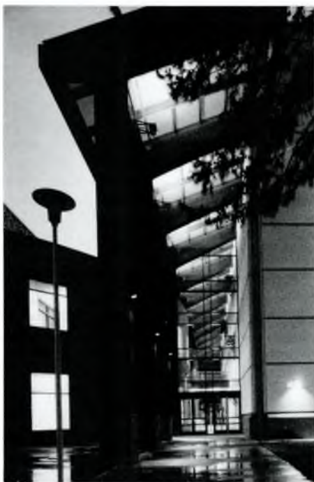
Cal State, Fullerton's new library addition offers seating for an additional 2,300 readers and nearly double the square footage.
