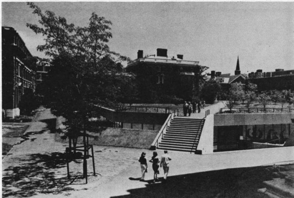
Pusey Library at Harvard: By placing the library below grade the buildings surrounding Harvard Yard remain unobstructed. (Photo: E. J. Jacoby).
