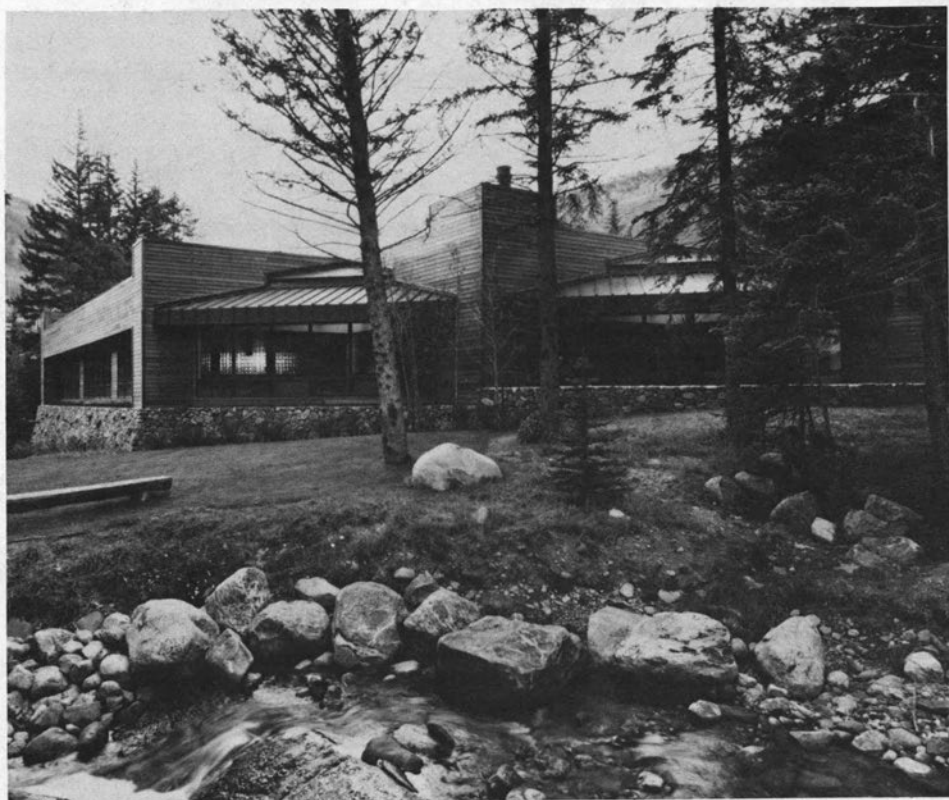
The Vail Public Library is recessed into a slope with a grass-lawn roof. (Photo: T. Hursley, Little Rock, Arkansas).
