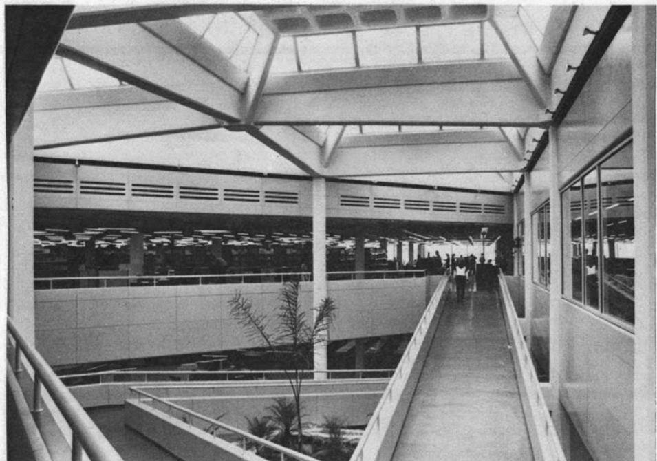
Gericke Library, University of Stellenbosch, South Africa: Visual emphasis is placed on the main circulation ramp in the atrium connecting both underground levels. (Photo: J. Stande, Stellenbosch).
