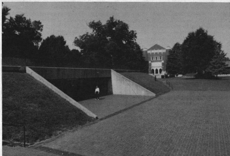
Hendrix College in Conway, Arkansas: Large sunken plaza is the approach to library's entrance. Earth removed from the plaza was used to bank library and landscape mall.
