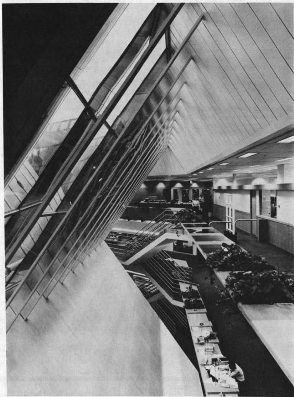
Law Library Addition, University of Michigan, Ann Arbor: A series of mirror mullions at left permit light to enter all levels which form balconies overlooking the light well.
